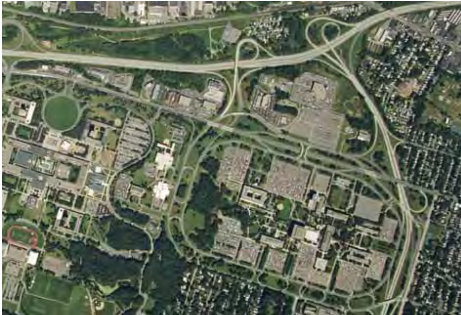
The 330 acre W. Averell Harriman State Office Campus is an unparalleled opportunity for redevelopment and reinvestment.
